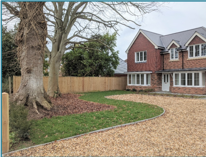
Figure 12. A new access and driveway situated in close proximity to protected, mature Oak and Beech trees through the use of a 3D cellular confinement-based surfacing system
