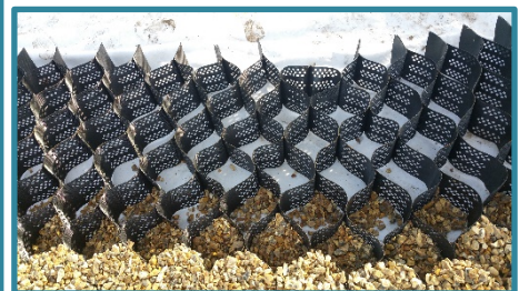
Figure 11. A cellular confinement system awaiting infill
