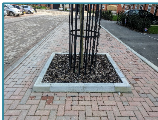
Figure 22. A well-executed tree planting within hardstanding
